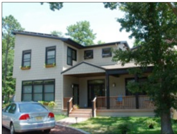
LEED Silver— net-zero electric energy home in Toms River, NJ.
